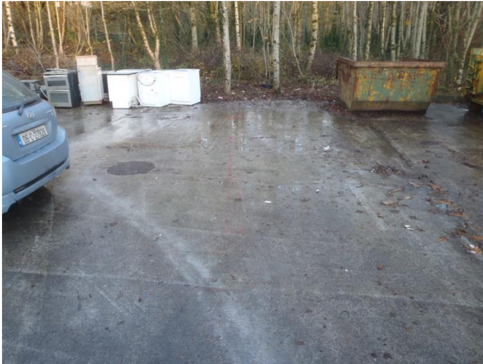
Photo 3: general view east from the lower yard area, with wooded copse area in the background. A foul sewer manhole is visible, with the septic tank located behind (beside white goods). Note the absence of kerbing at the edge of the concrete pad beside the white goods.
