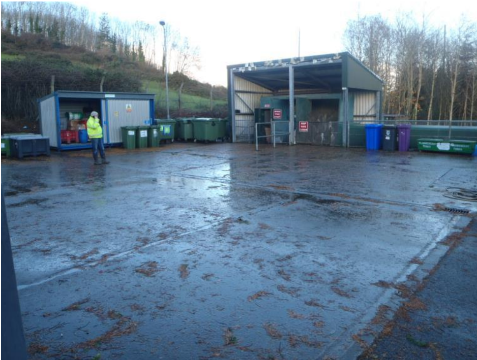
Photo 1: general view of upper yard area.
