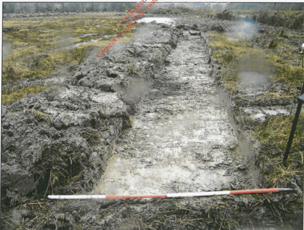
Plate 8: Trench 24, facing north – note very wet and disturbed area north of trench
