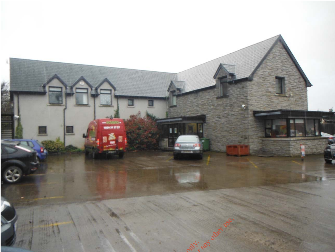
Figure 1.3: Yard Area Front of Office
