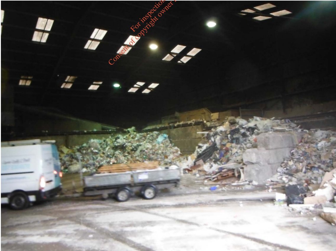
Figure 1.16: MRF: Skip & MDR Tipping Area
