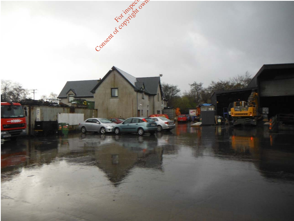
Figure 1.6: Yard Area: Rear of Office
