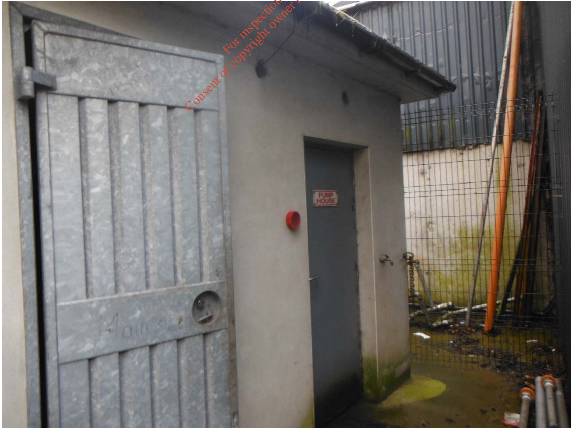
Figure 1.26: Yard Area: Emergency Key for Pump House
