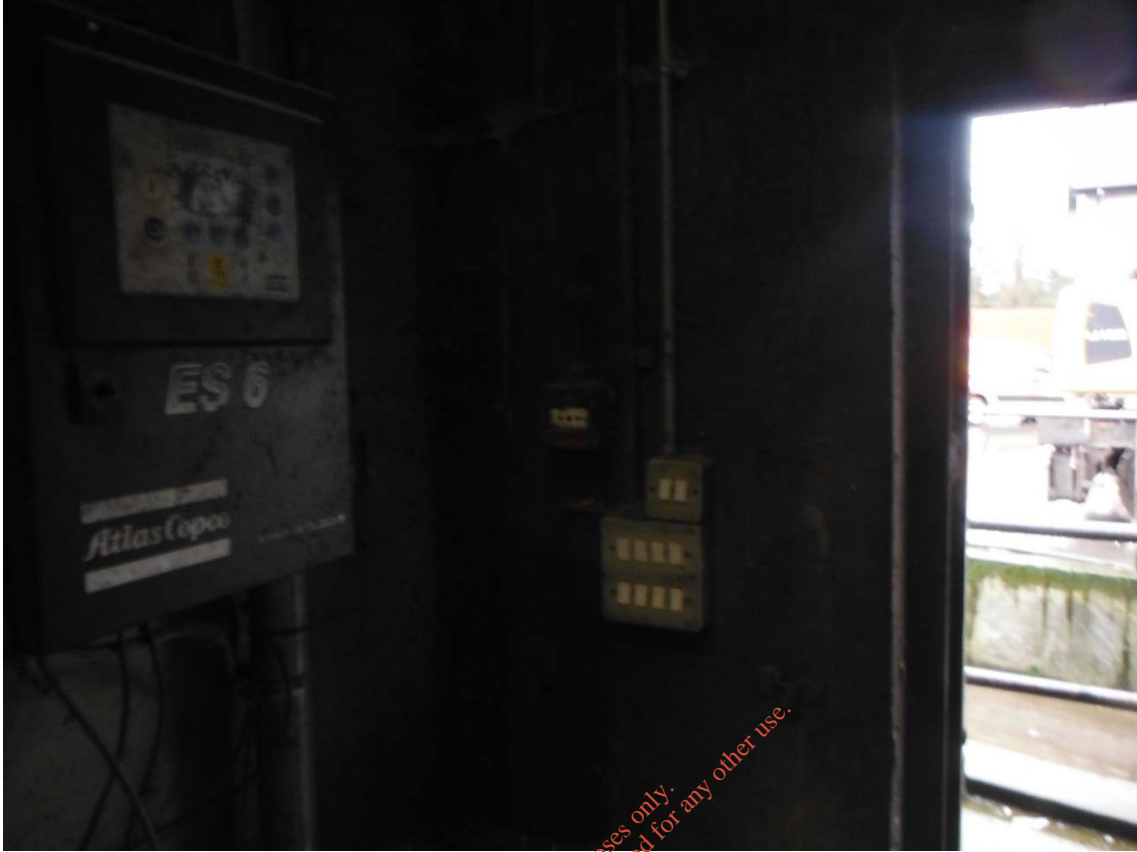
Figure 1.21: MRF: Break Glass Alarm Unit
