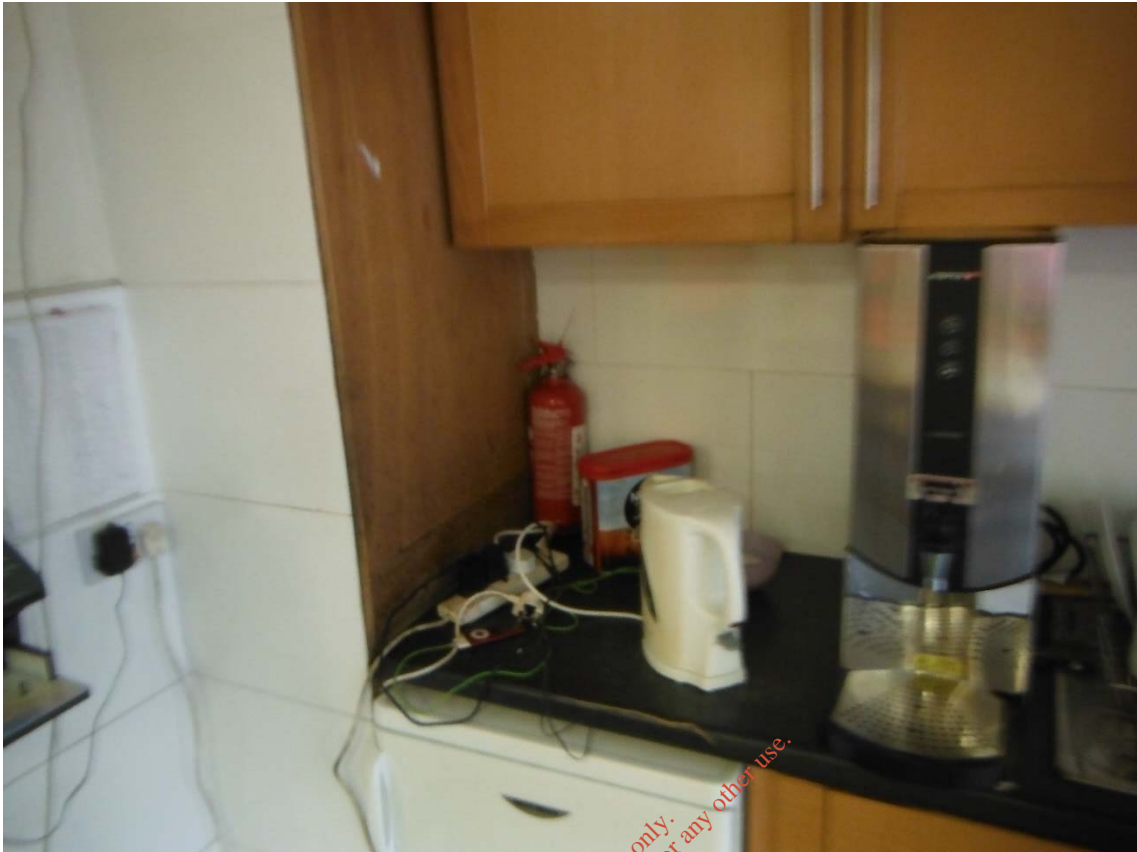
Figure 1.29: Office Building: Fire Extinguisher in Canteen
