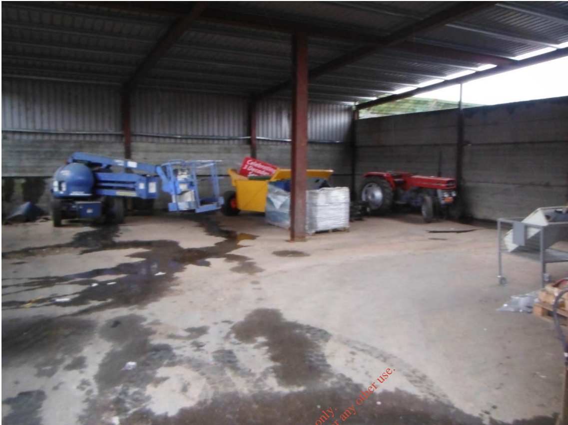
Figure 1.9: Plant Storage Shed (previously bailed plastic shed)
