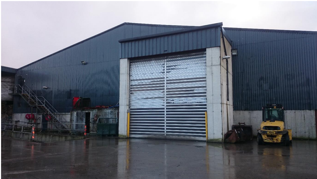
Photograph 1 Main Processing Building
