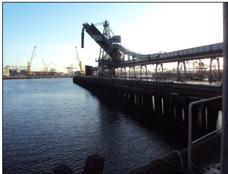
Plate 3.2 View of the Bulk Jetty
