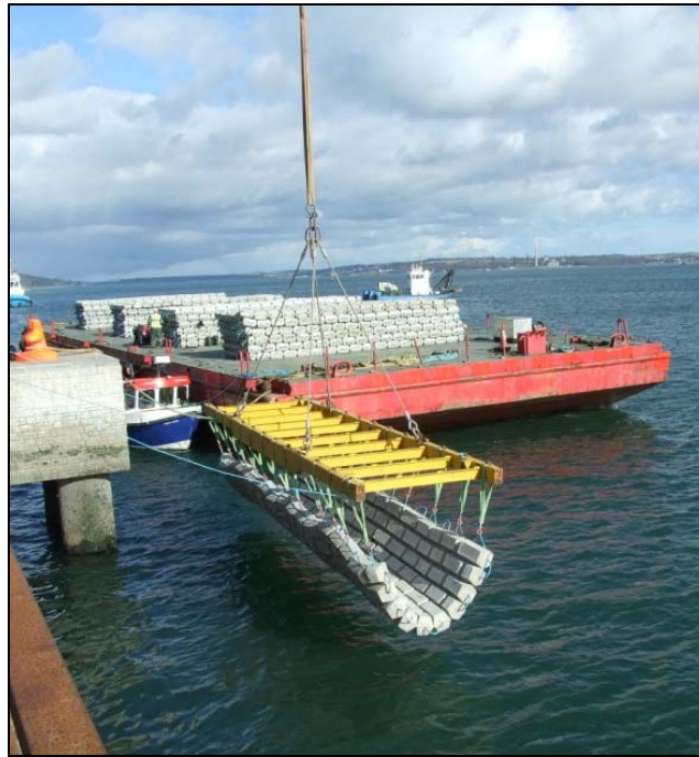
Plate 4.2 Concrete Mattresses being Lifted into Position
