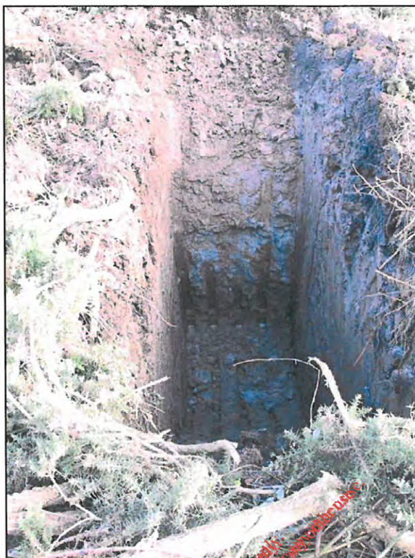
Plate 7: Section from Trial Pit 7
