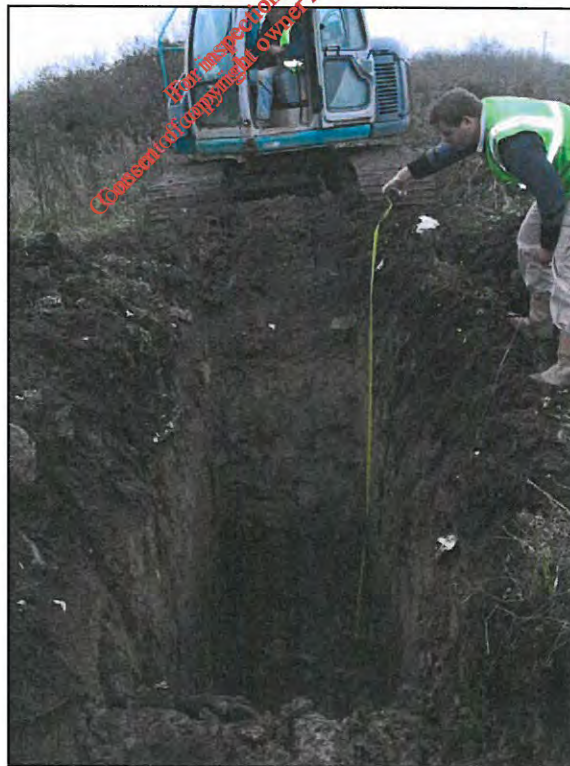
Plate 2: Section View of Trial Pit 2
