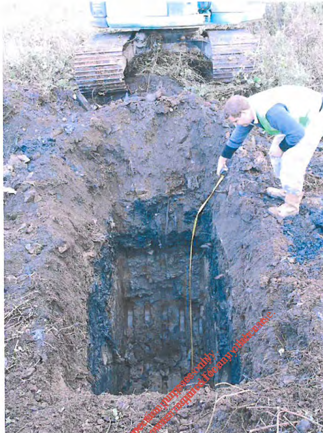
Plate 3: Section View of Trial Pit 3 – note thin layer of black fill material (c.0.5m)
