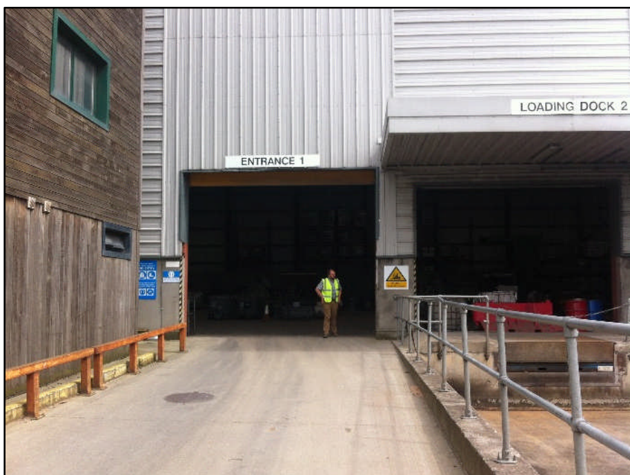
Figure 1: Warehouse/transfer station entrance for designated waste residue transfer area (external view)
