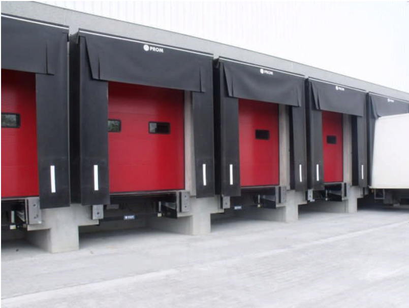
Figure 10: Loading bay seal for safe loading
