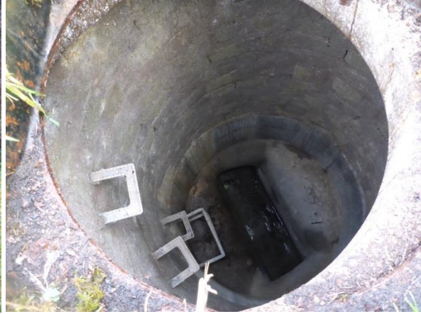
Image 2: Sewer adjacent to SW003 location
