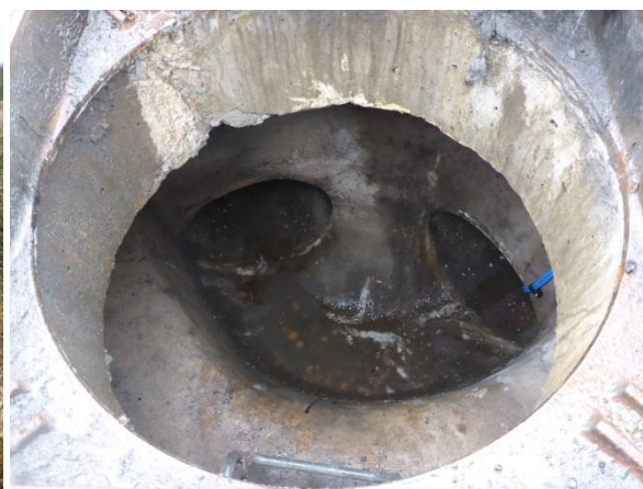
Image 6: Last manhole before SW005
