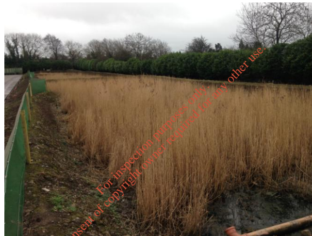
Reed bed used for surface water treatment
