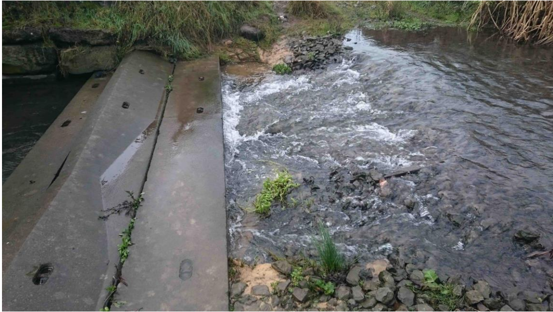
Plate 3 Tramore River: Site C – showing undercut crump weir (22-12-2016).
