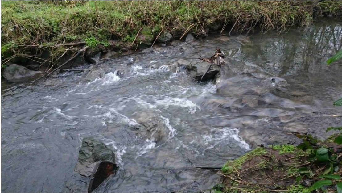
Plate 5 Tramore River: Site D – showing natural cobble boulder weirs just above which kick samples were taken (22-12-2016).
