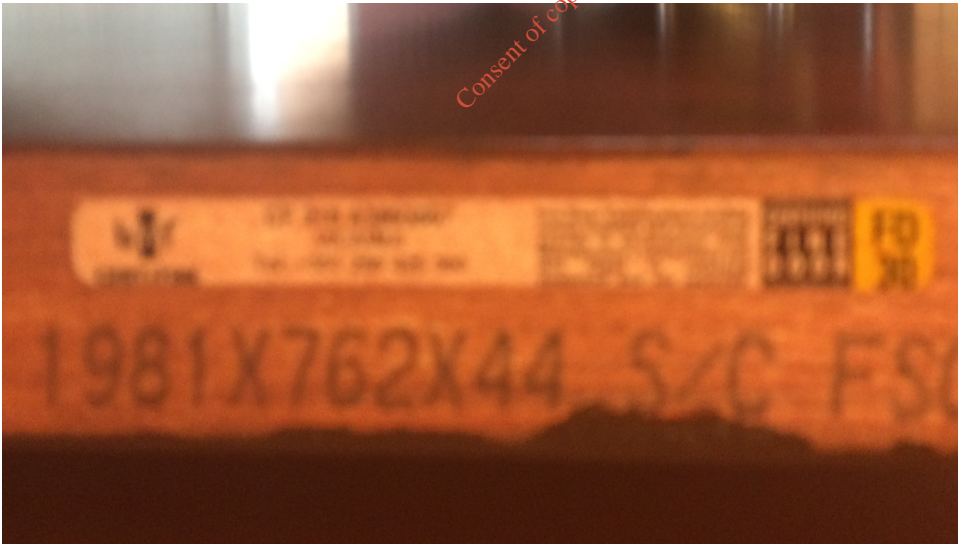
Figure 18 Item 3.2.3 FD30s Fire Doorsets installed.
