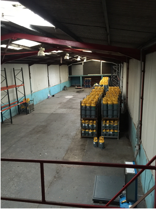
Figure 11: No Emergency Lighting
