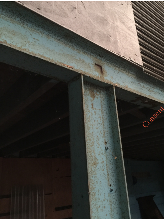
Figure 16: Column and Beam supporting Mezzanine
