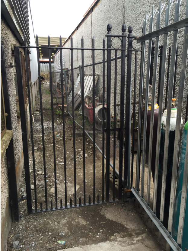
Figure 17 Item 3.1.4 Gate and route to gate cleared.
