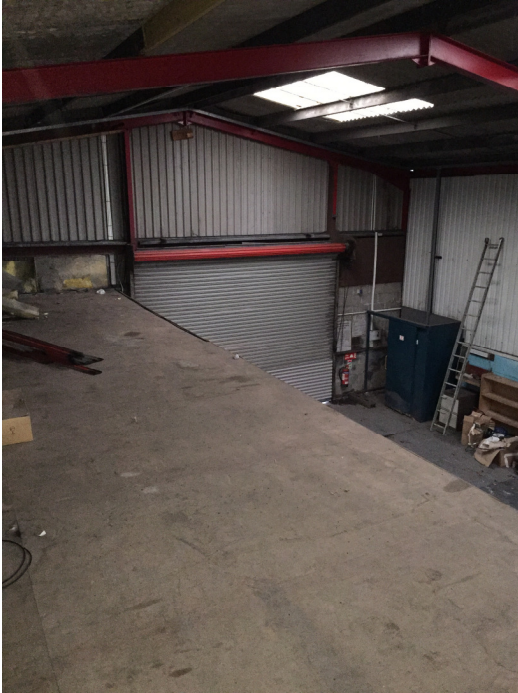
Figure 9: View from front mezzanine
