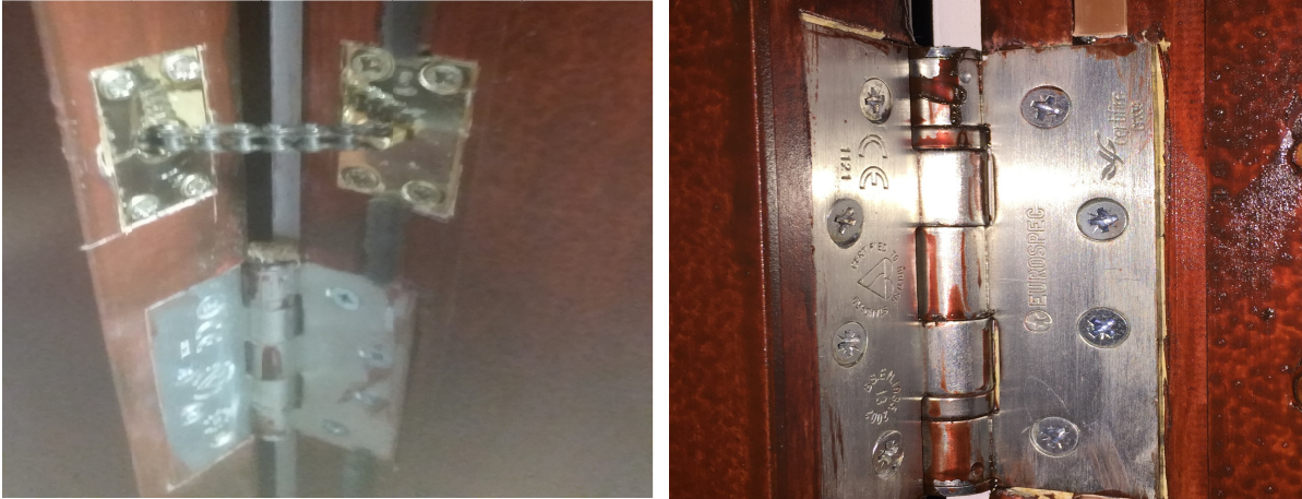
Figure 19 20 Item 3.2.3 FD30s Fire Doorsets installed.
