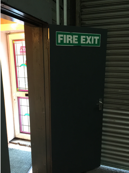
Figure 7: Door from Main hall to Main Entrance
