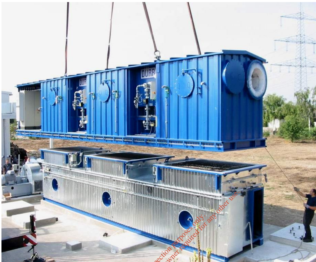
Components delivered as pre-assembled sections for fast installation
