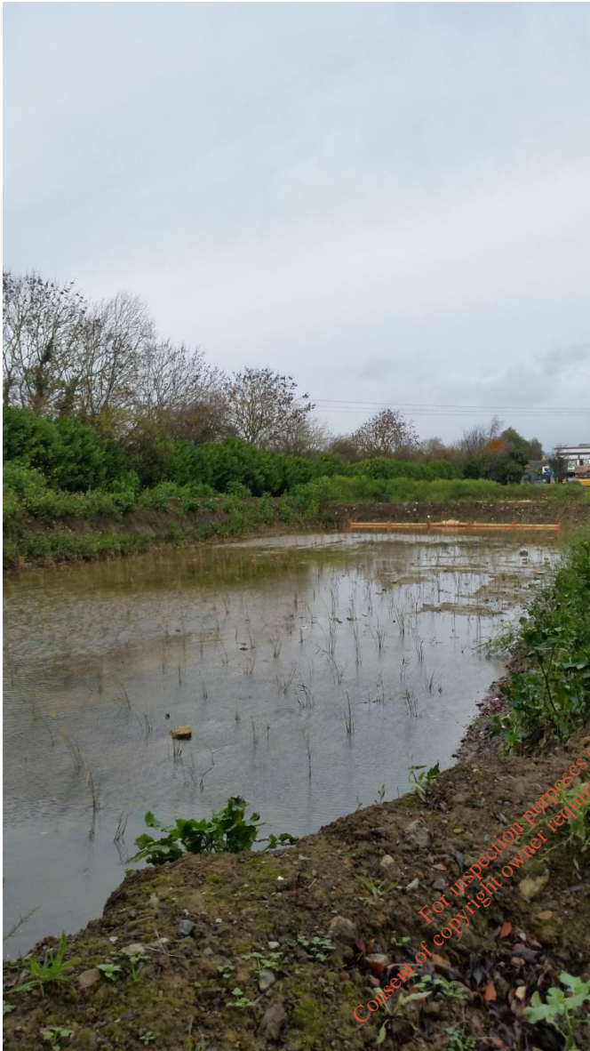
Photo 1 showing newly constructed wetland.
