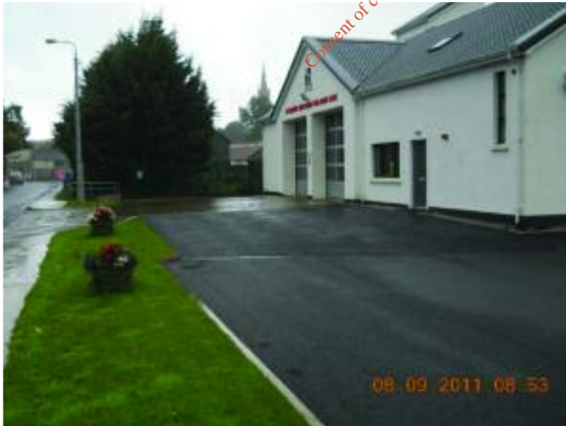
Clones Fire Station (on 98 Avenue) situated on raised land, but access is onto the flooded 98 Avenue.
