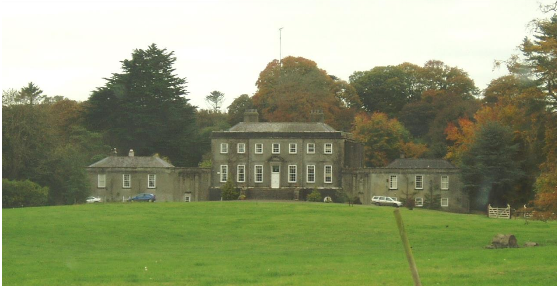
Plate 11-1 View of Swainstown House
