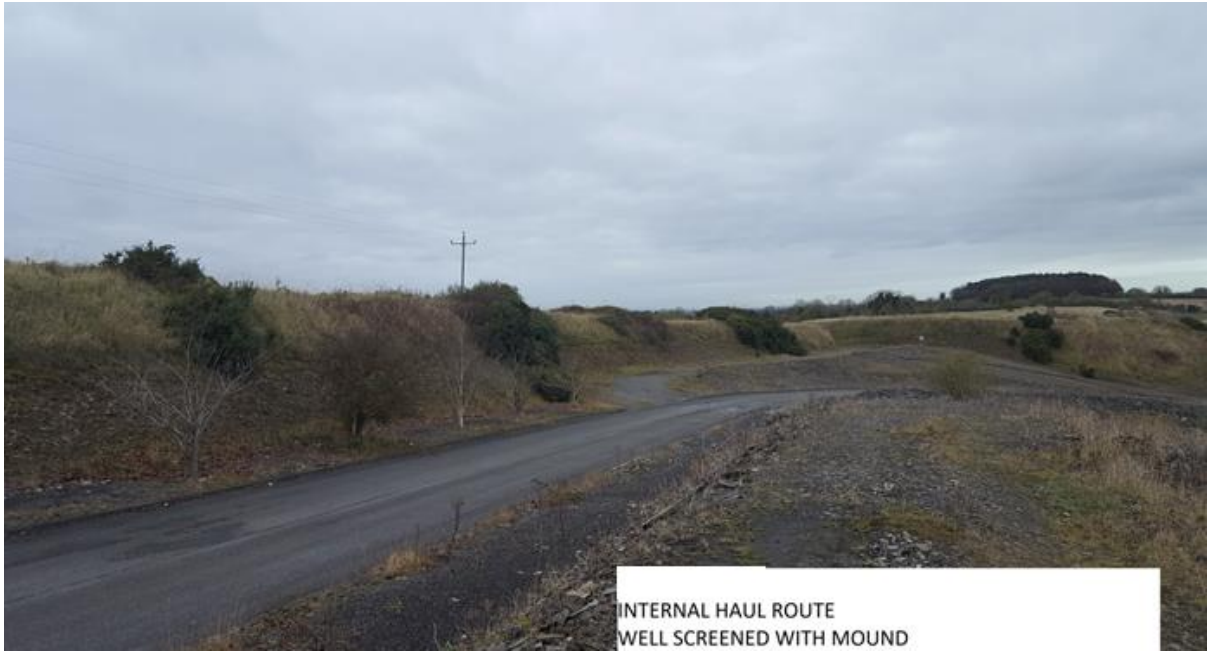
Plate No 10: Internal Haul Route with visible screening mounds
