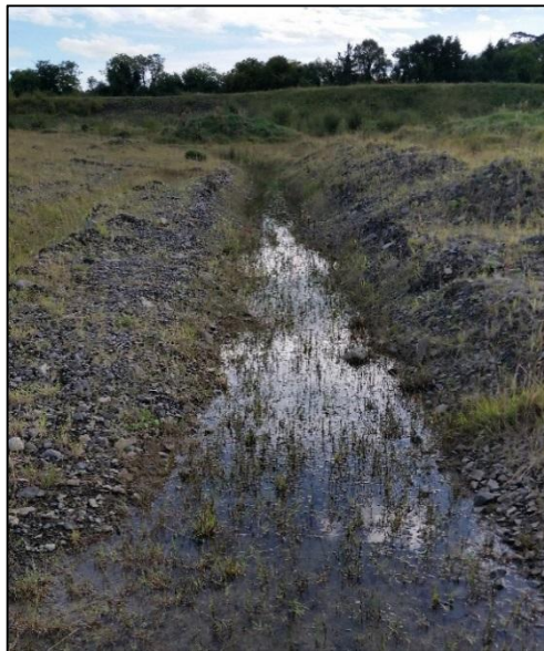
Plate 10: Drainage ditch (FW4) located within the eastern section of the subject lands, surrounded by recolonising bare ground (ED3) habitat type. Photograph taken facing a southerly direction.
