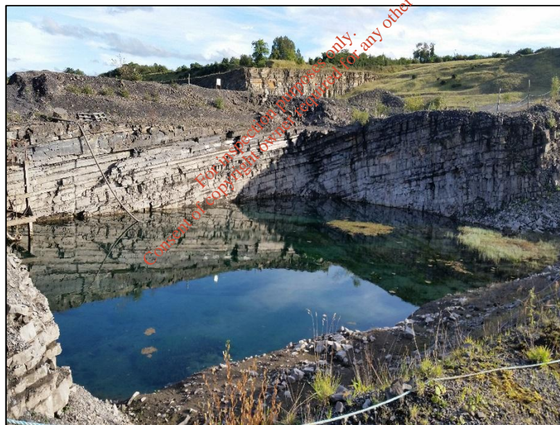
Plate 8.2: Sump located within the centre of the quarry floor. Photograph taken facing a south-easterly direction.
