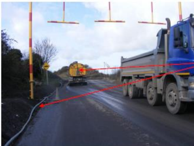
Plate 2 – Road Sweeper and Sprinklers under Construction
