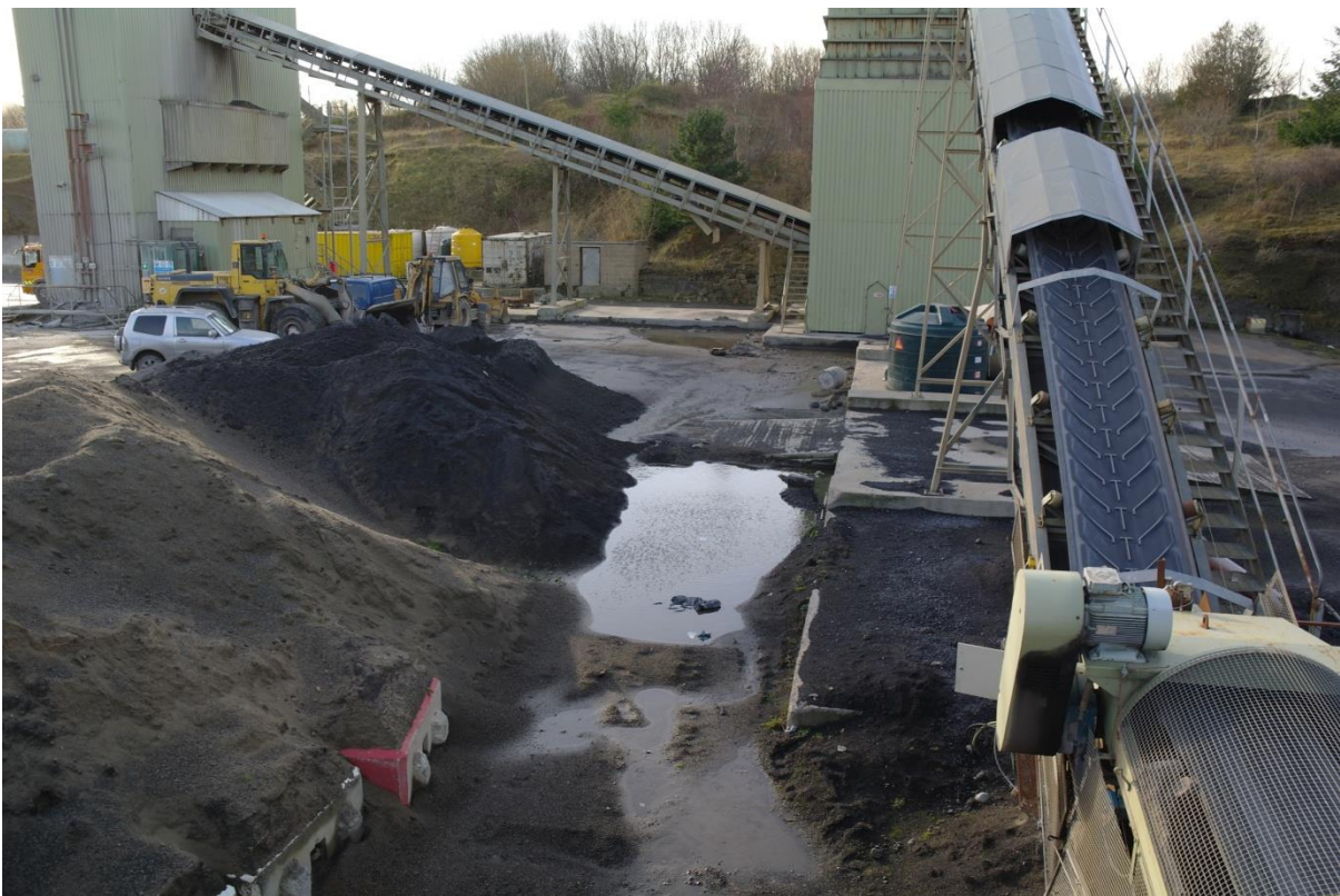
Photo 5 – Yard Drainage Impeded by Concrete Platform
