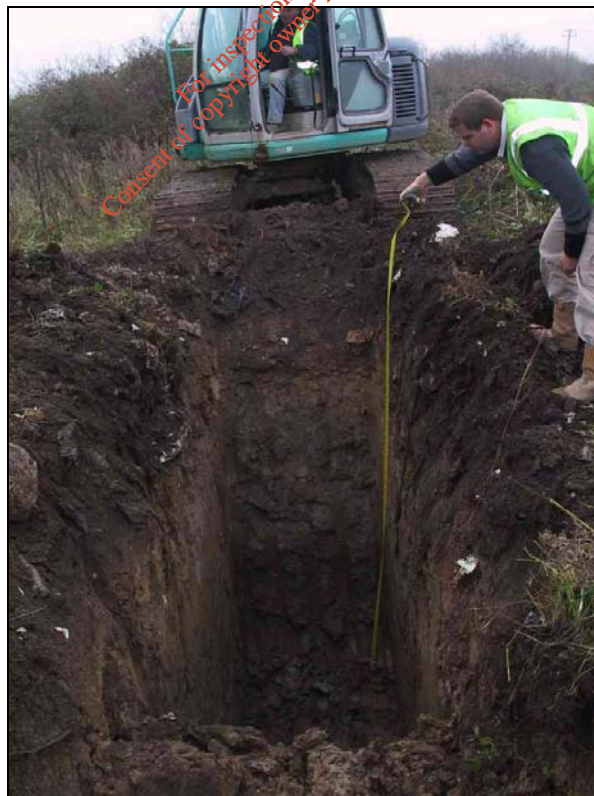
Plate 2: Section View of Trial Pit 2
