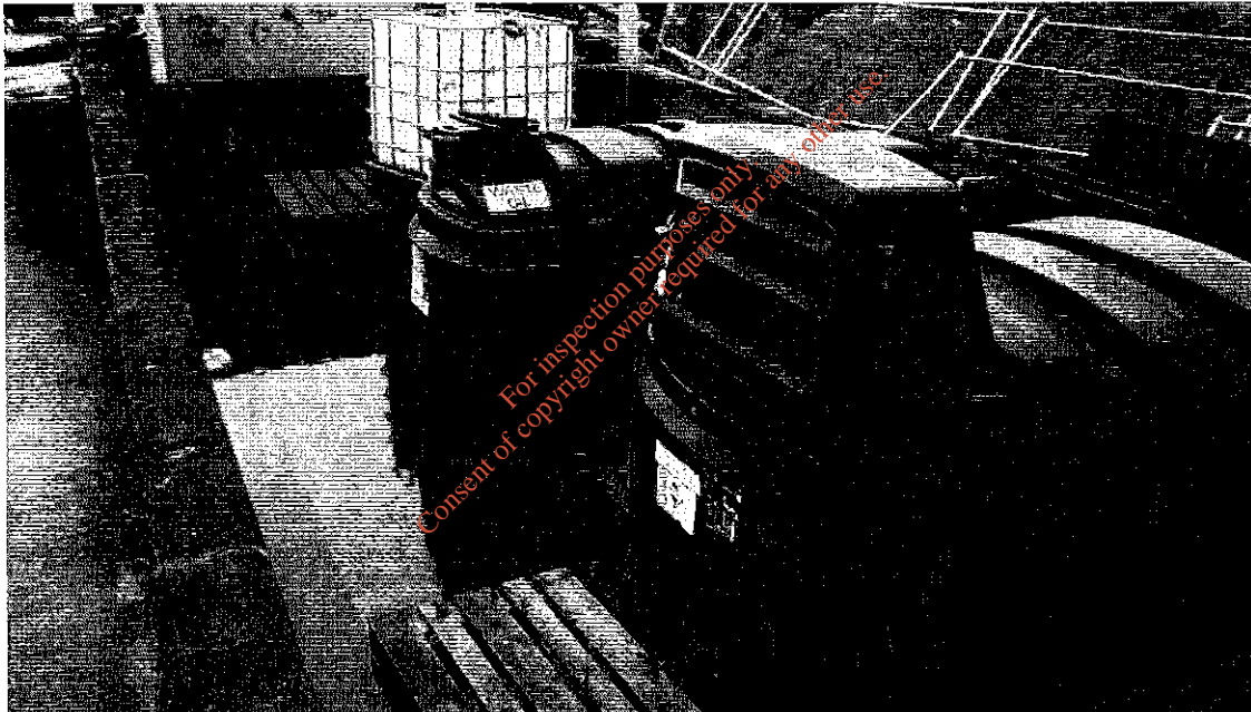
Photo 2 – Green Diesel and Waste Oil Tanks
