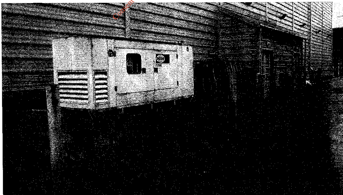
Photo 3 – Diesel Tank at Back-Up Generator
