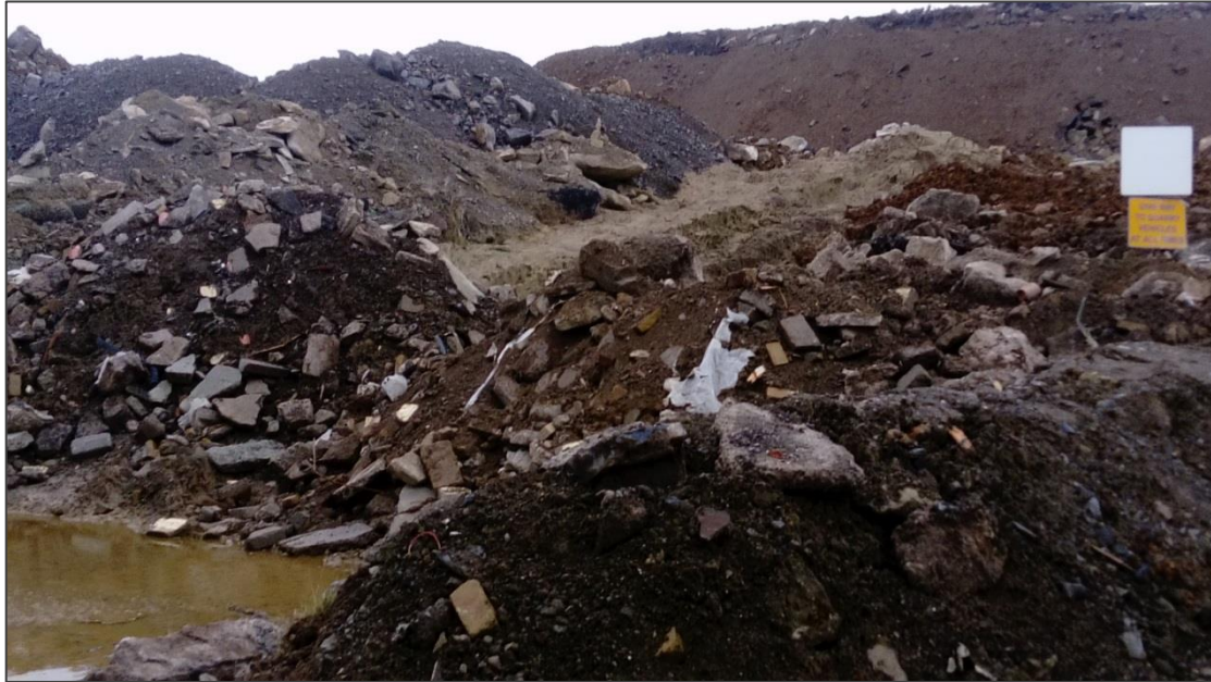
Figure 3: Stockpiles of C&D waste in the fill area
