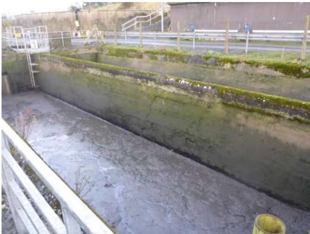
Photo 3 – 58m 3 storm water holding tank (2 compartments)
