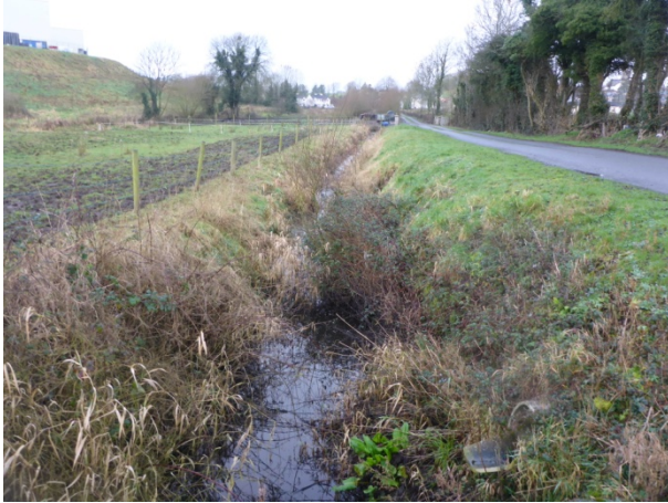
Photo 2 – SW003 adjacent prior to the WWTP inlet works
