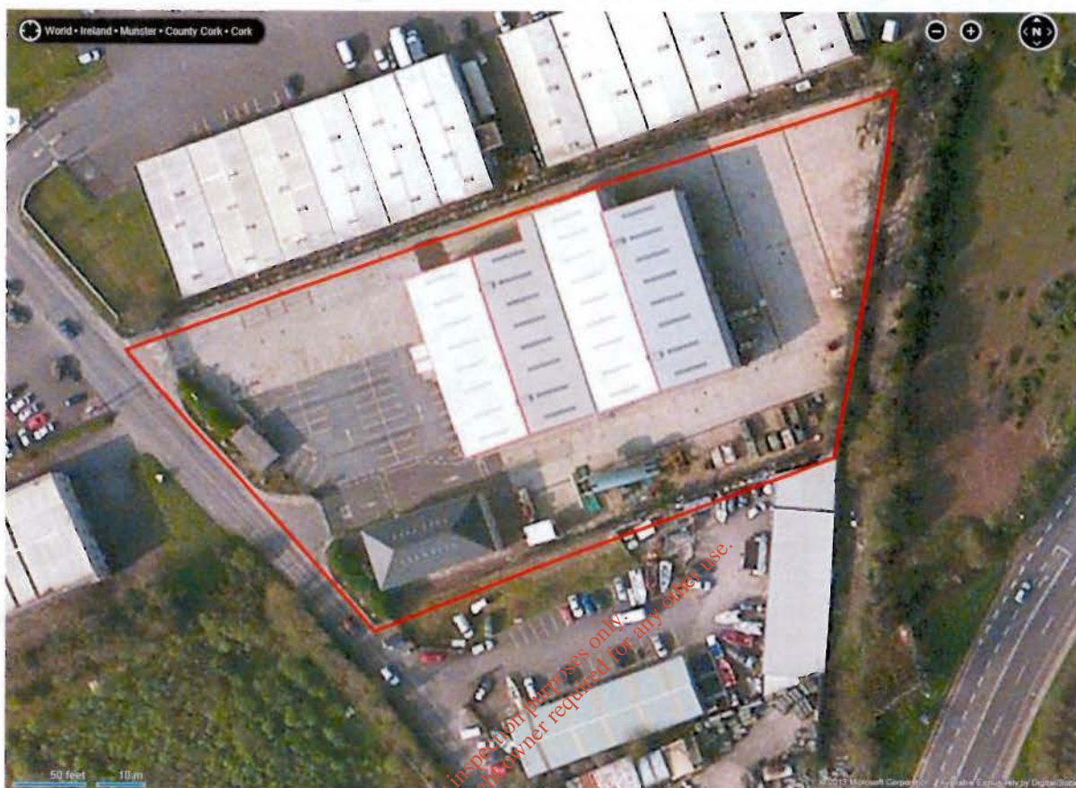
Figure A.1.2 – Aerial View of Site
