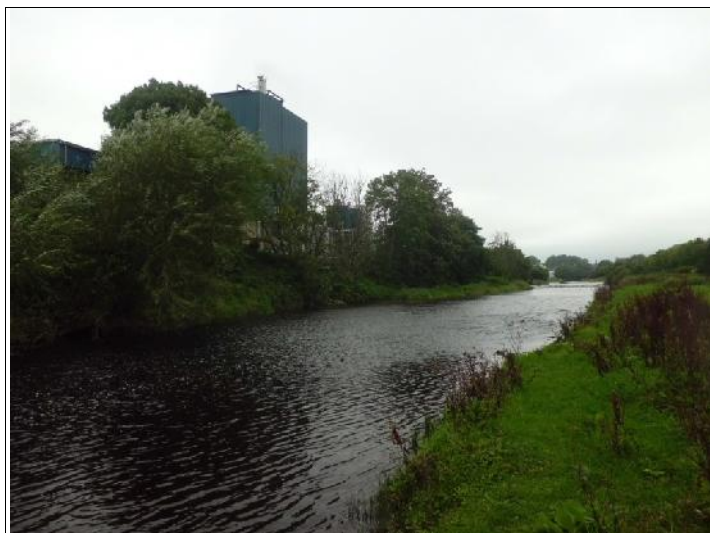
Figure 11.3 The banks of the River Allow looking N from the E bank; the site under review is on the W bank
