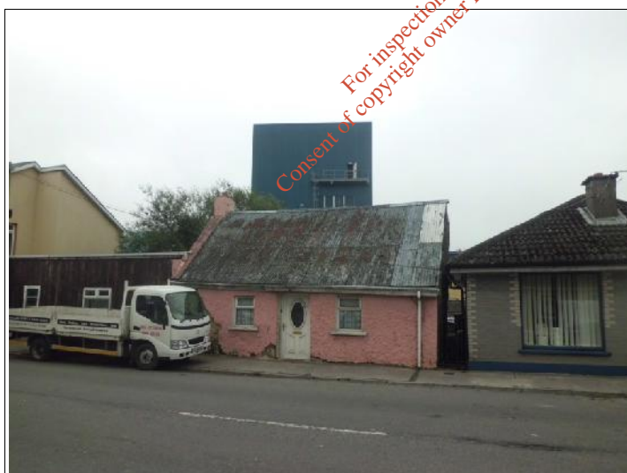
Figure 11.12 On the S side of Bluepool Lower only one of the original cottages survive in a form close to the original (the house may once have been thatched). Most of the cottages have been replaced with modern houses and the complex of modern co-operative buildings can be seen in the background.
