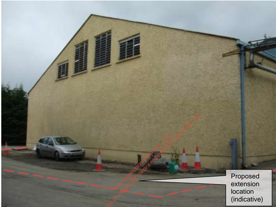
Figure 3-2 Existing Casein Plant building, showing approximate location of proposed extension
