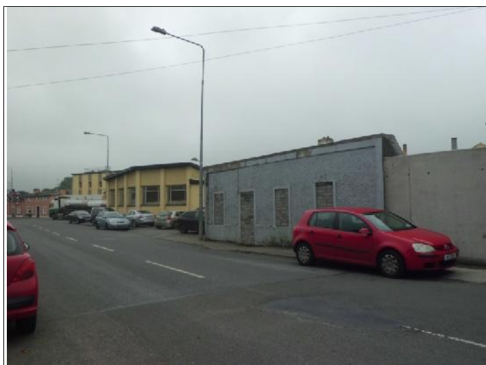
Figure 11.11 Some of the former houses on Bluepool Lower are represented by only the front walls. While the 1950's style creamery buildings can be seen in the background.
