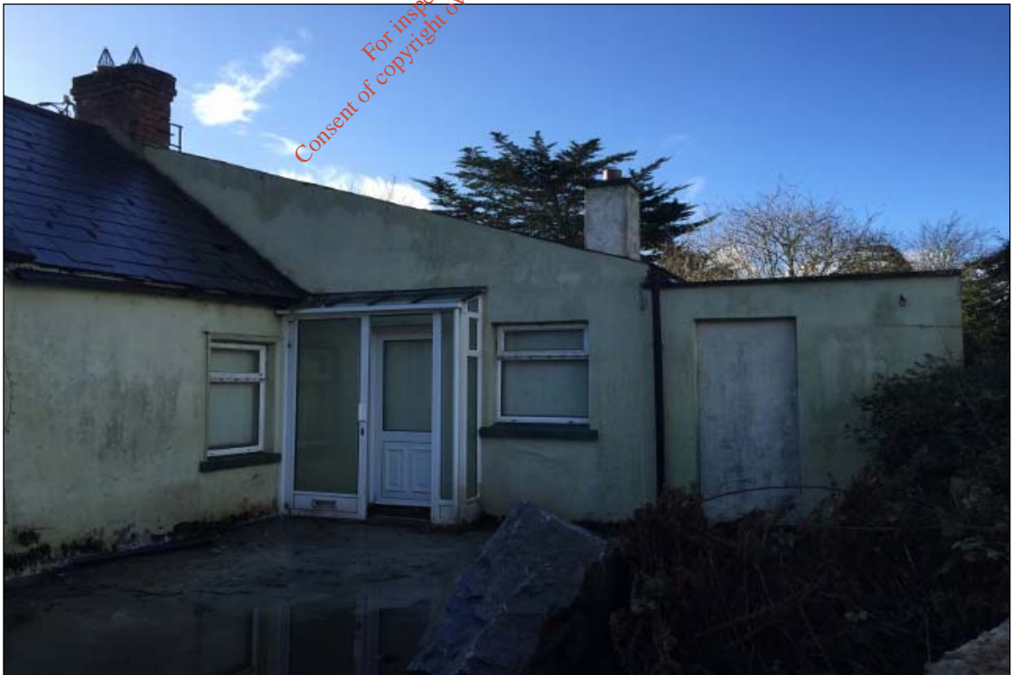
Plate 2: Disused cottage adjacent to the bungalow in Plate 1 above
