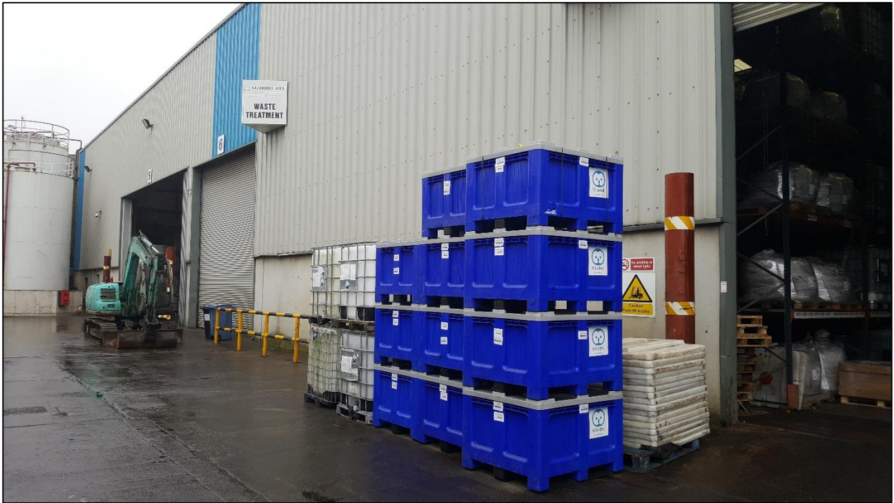
Figure 1: Waste transfer building entrance for bagging and transfer of ash waste residues (external view)
