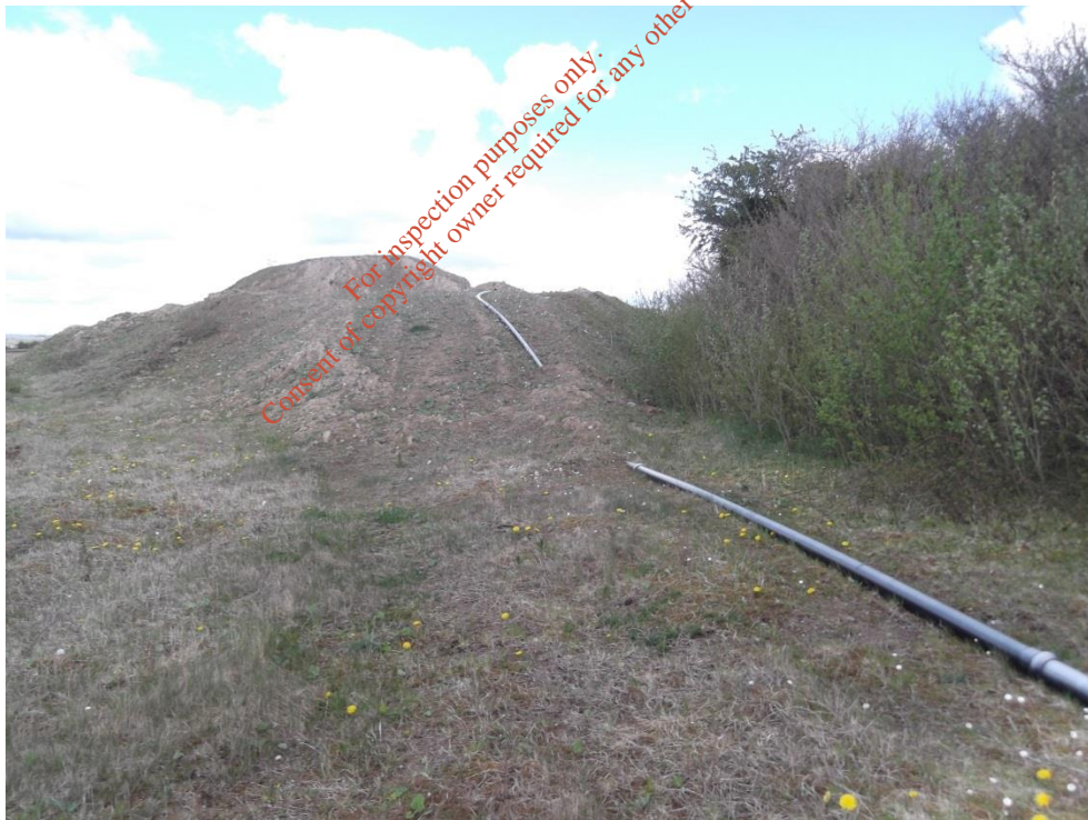
Plate CH-3 Silt Pond Retention Bund located close to north-western corner of SITE CH-1 (looking north)
