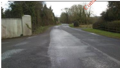
Photograph 1.0: Southbound view into R401 from existing gravel pit access.
