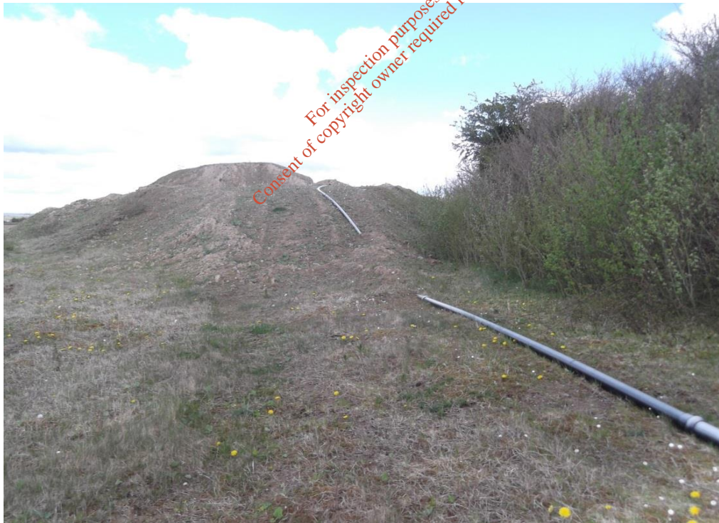
Plate CH-3 Silt Pond Retention Bund located close to north-western corner of SITE CH-1 (looking north)
