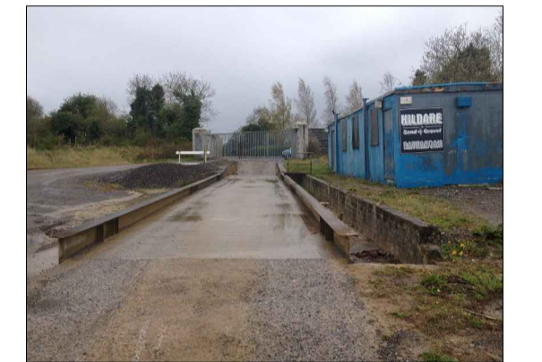
Existing Weighbridge & Wheel wash
