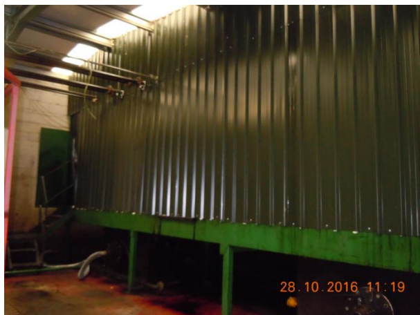
Figure 15 New screening partition (left photo) separating the oil filtration plant (which is located behind the partition) from the remainder of the treatment building (which currently contains centrifuges and heat exchangers and will, if it's installed, contain elements of the flash distillation plant). The area behind the wall is mechanically ventilated and off-gases are treated in a carbon filter (right photo). The vertical orange pipe is the feed into the base of the carbon filter. The emission point is at the top.
