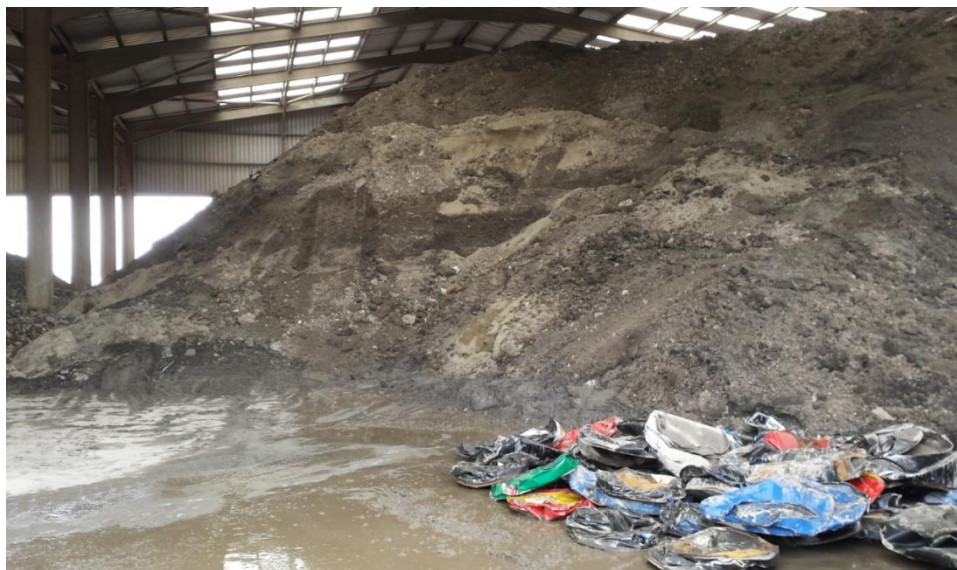
Figure 4 The interior of the waste soil treatment building, not fully enclosed at time of photo (February 2016)
