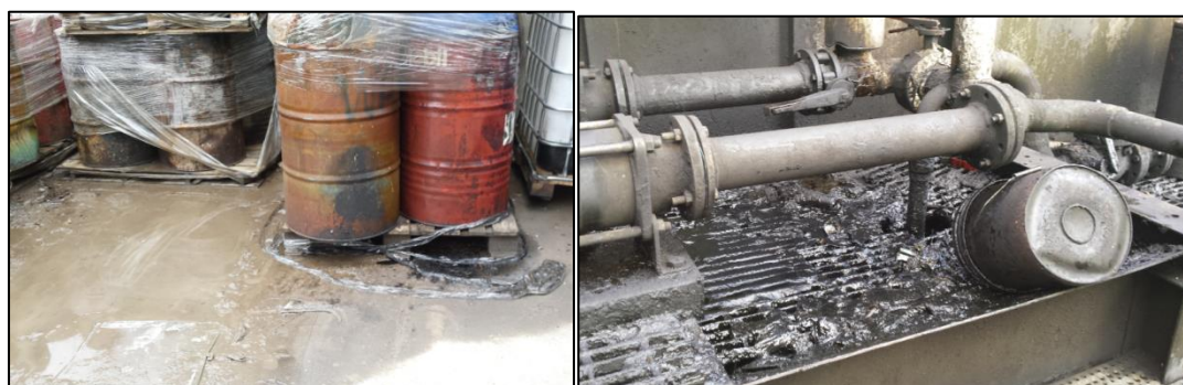
Figure 10 Photos (February 2016) showing potential sources of stormwater contamination, namely from left, storage of dirty drums outdoors, a pump bund
