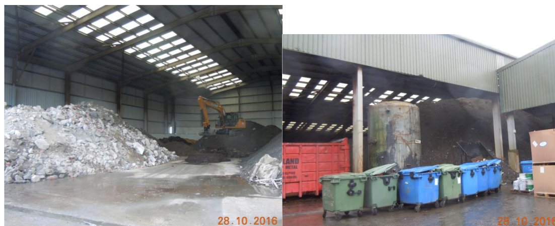
Figure 5 The interior of the soil treatment building (October 2016). The left photo shows the inside of the enclosure of the north and east facades. The right photo shows the south facade unenclosed and also shows some overspill of waste soil and the storage of waste containers out of doors. The west facade, not shown, is not enclosed.
