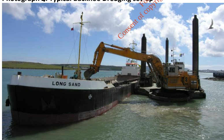
Photograph 4: Typical Backhoe Dredging set-up
