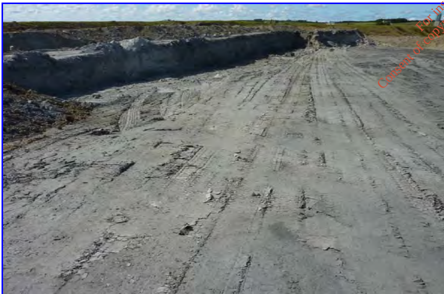
Figure 8.9: Example of initial stages of filling in ash storage area
