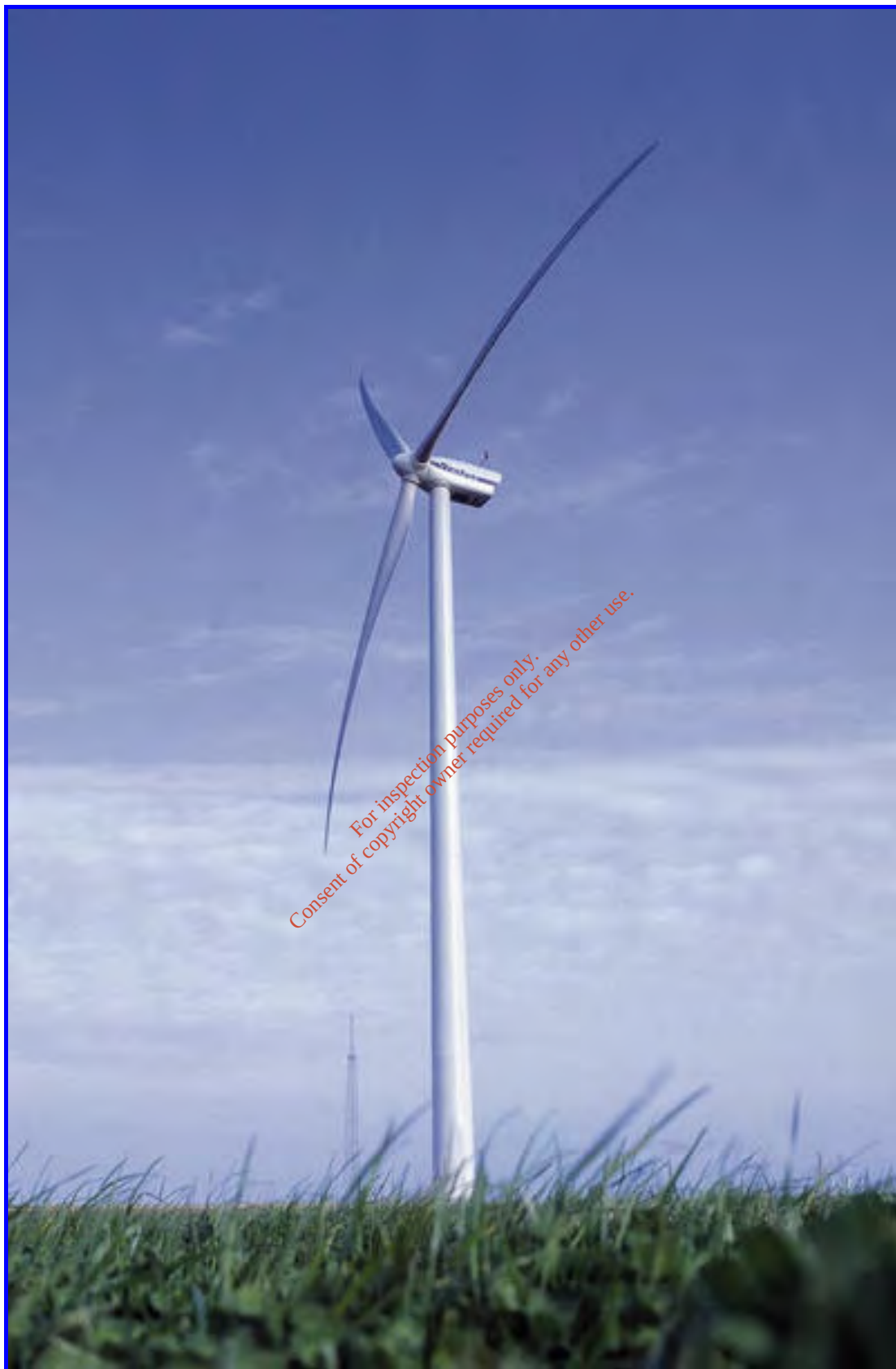
Figure 2.2: View of Wind Turbine
