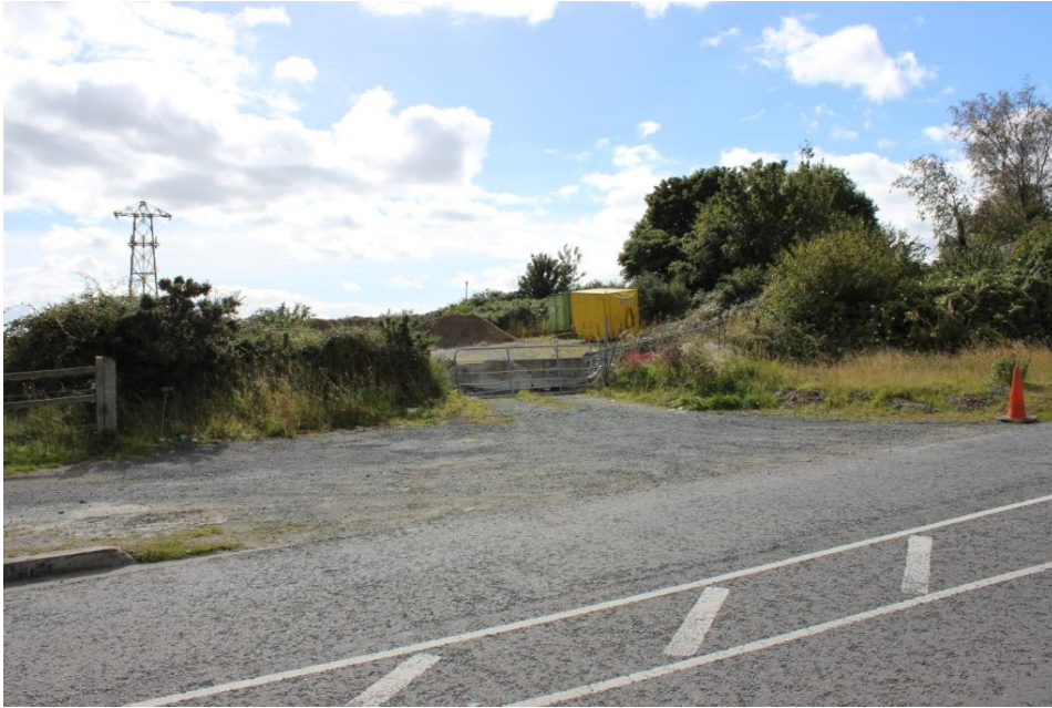
Figure 9-2: Main Existing Site Entrance
