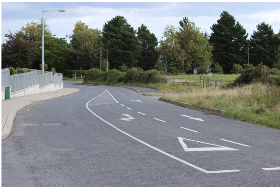
Figure 9-3: Main Existing Site Entrance (viewed from entrance to Farrankelly Close)
