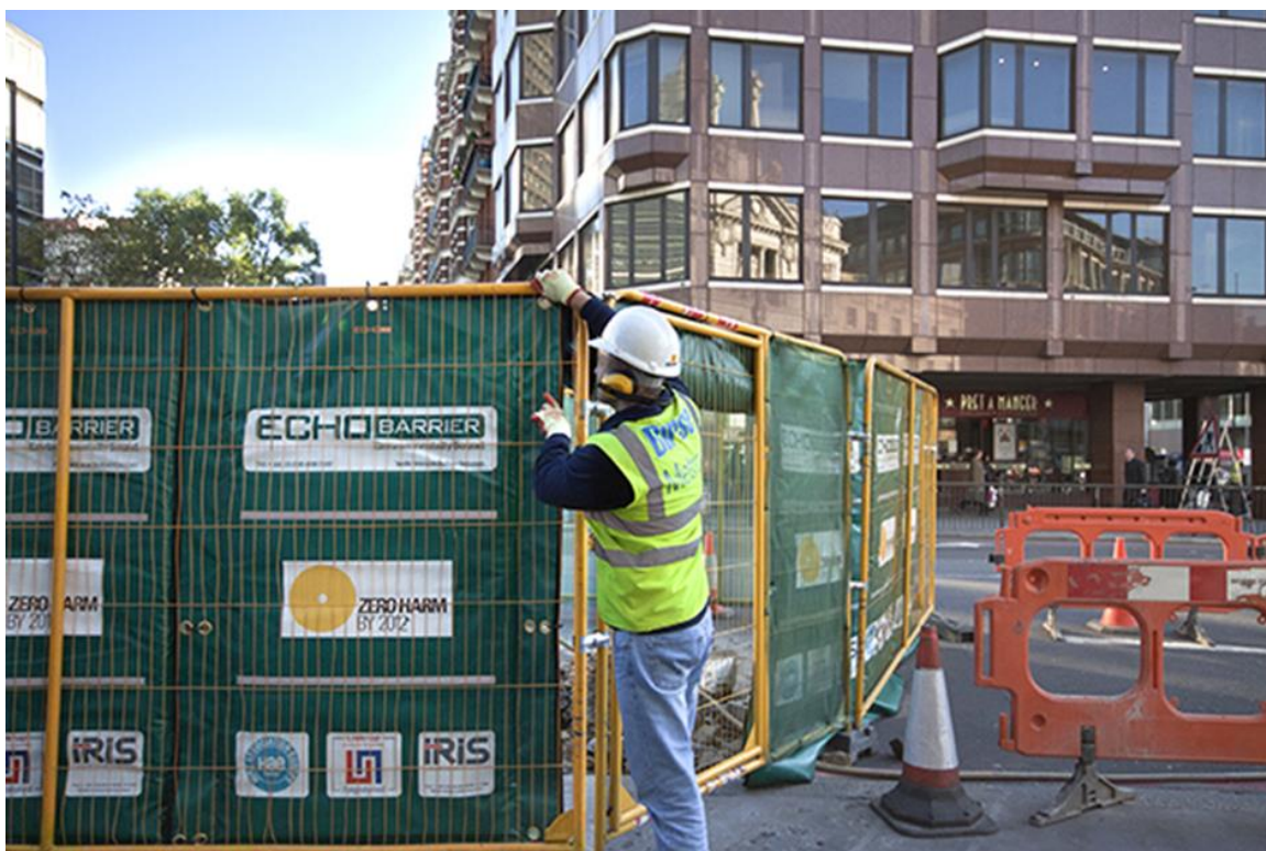
Figure 10-2 Example of construction acoustic fencing 34
