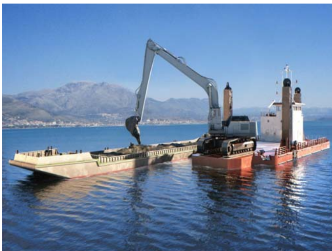
Plate 3.2 Mechanical Excavator on Floating Plant
