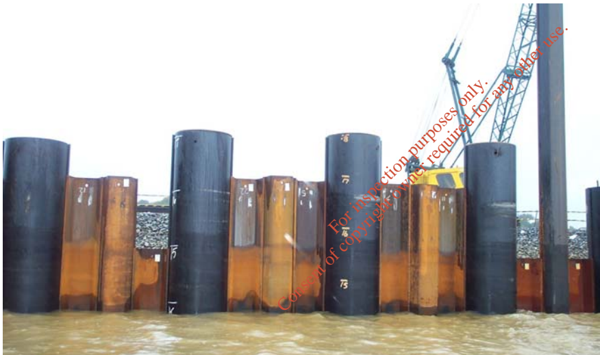
Plate 3.1 Example of Combi-wall Under Construction
