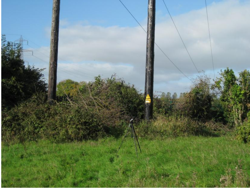
Noise monitoring equipment at monitoring location N3
