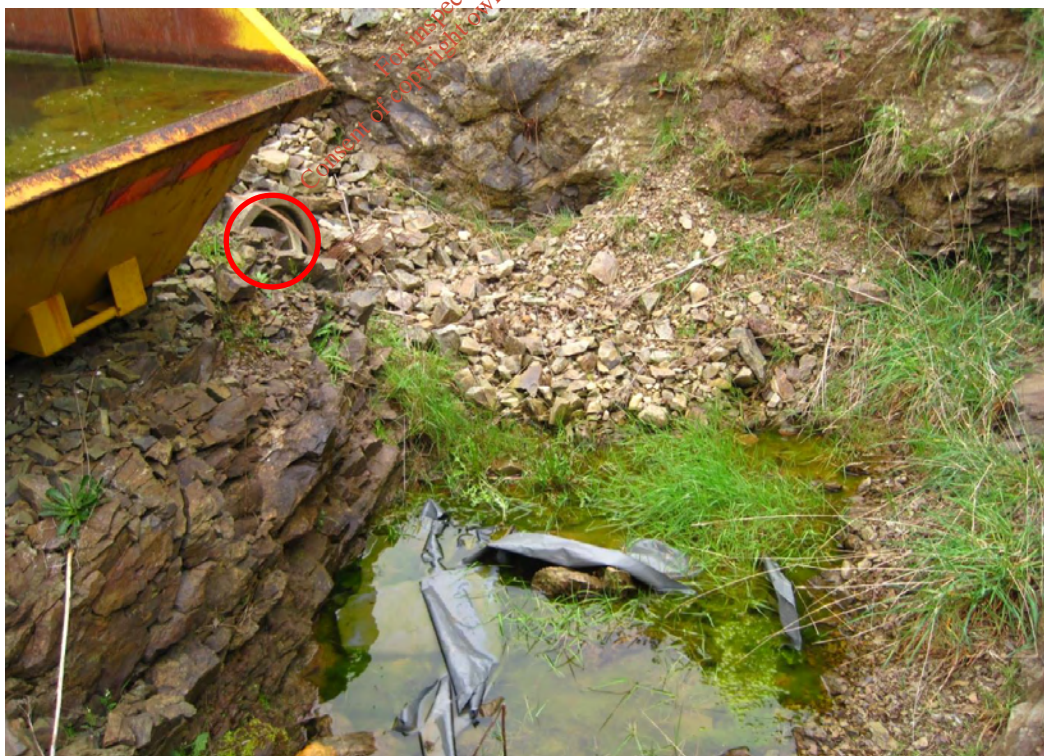
Plate 6-4 Existing High Level Sump and Discharge Pipe
