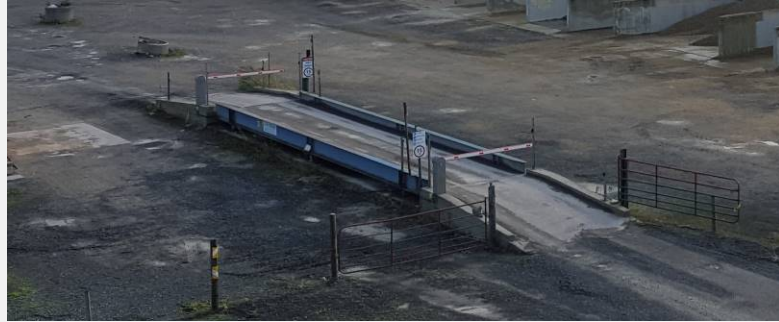
Existing Weighbridge & Barriers
