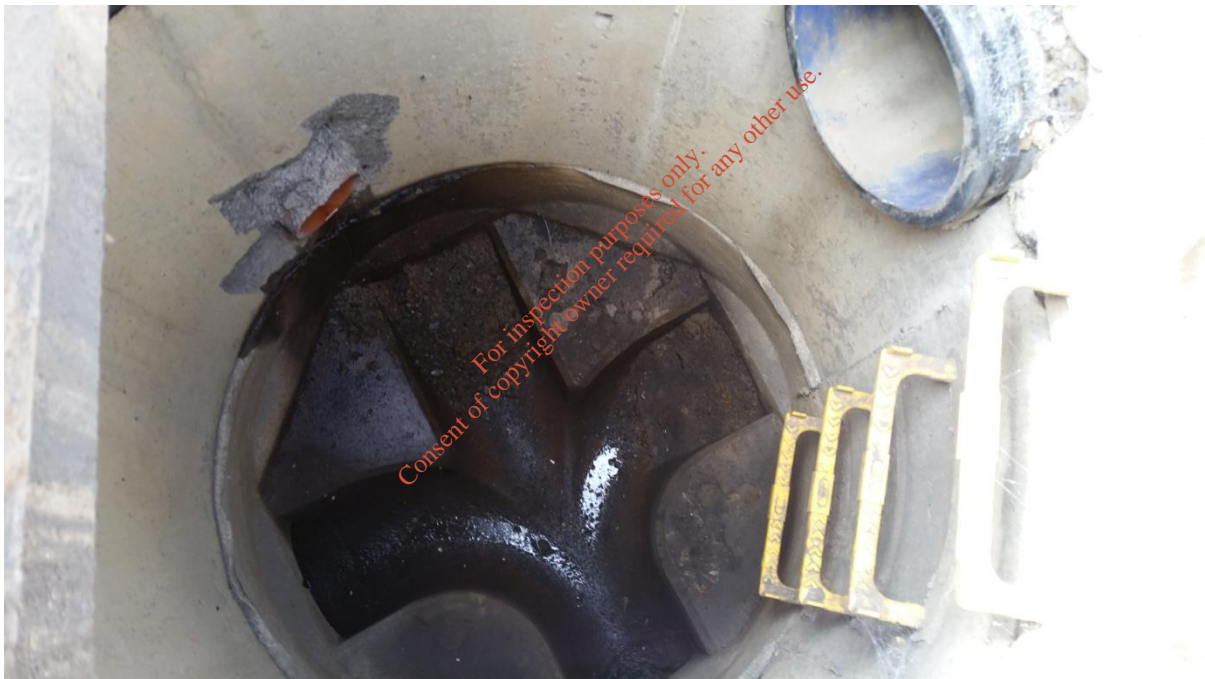
Photo D.1.6 – High Level overflow to Stormwater Discharge Point (SW1)
