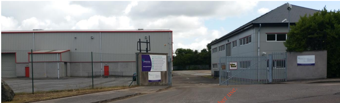
Photo D.1.1 – Southernmost Entrance Gate
