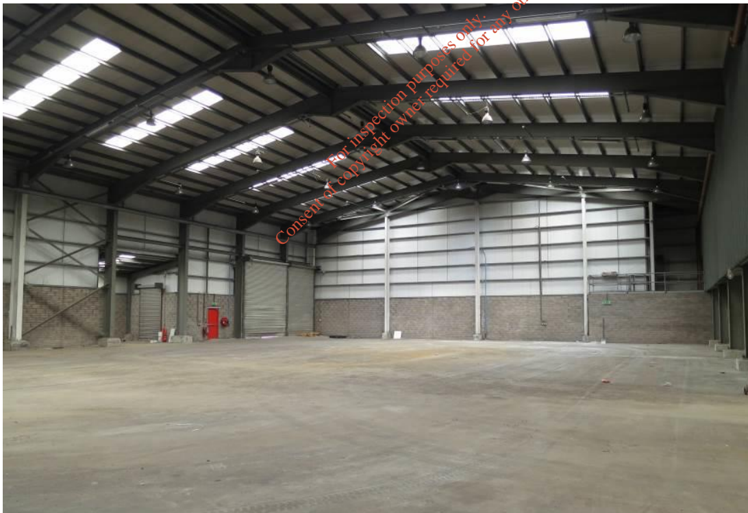
Photo D.1.11 – Internal view of Building 1
