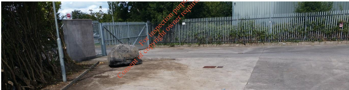
Photo D.1.2 – Northernmost Entrance Gate
