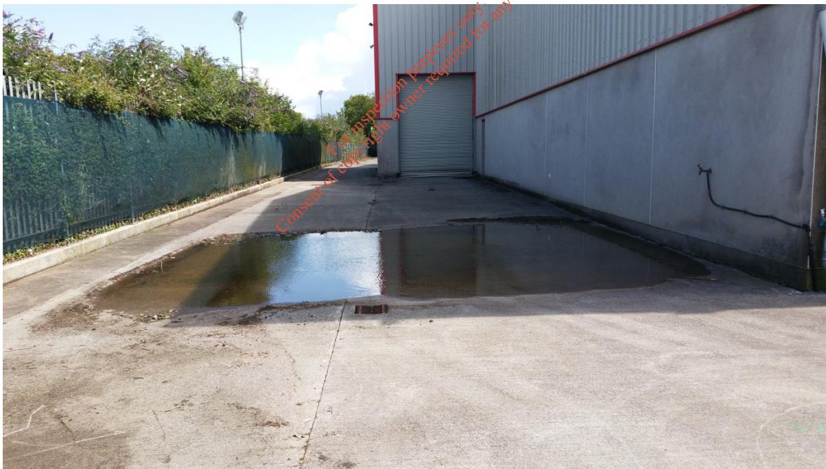
Photo D.1.3 – Existing Wheelwash
