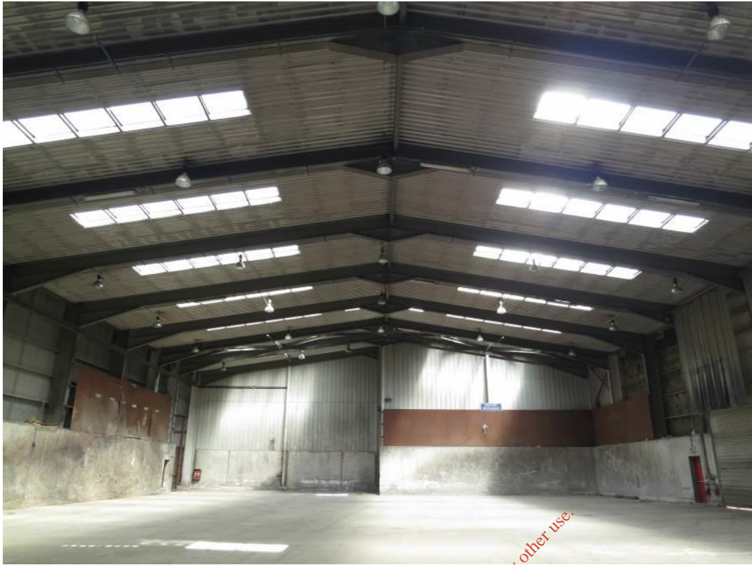
Photo D.1.12 – Internal view of Building 2
