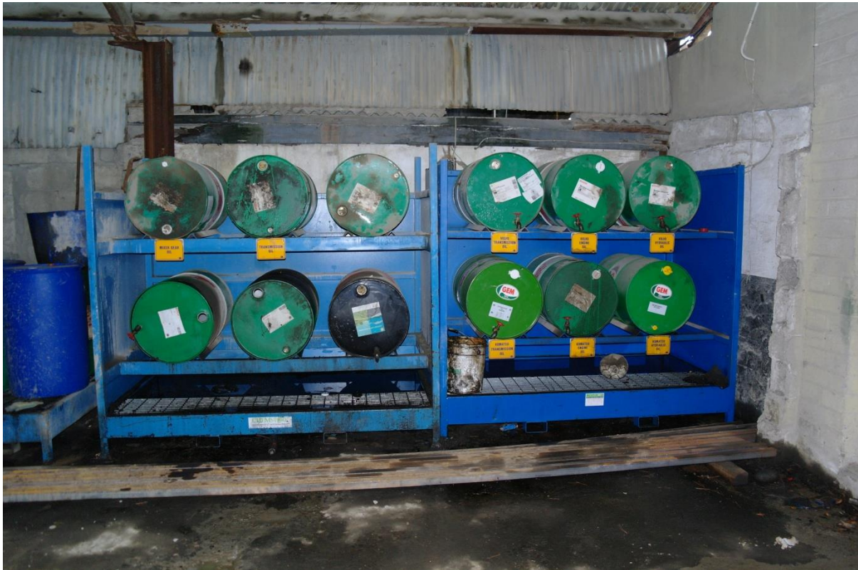
Photo 2 – Bunded Oil Drums in Maintenance Shed
