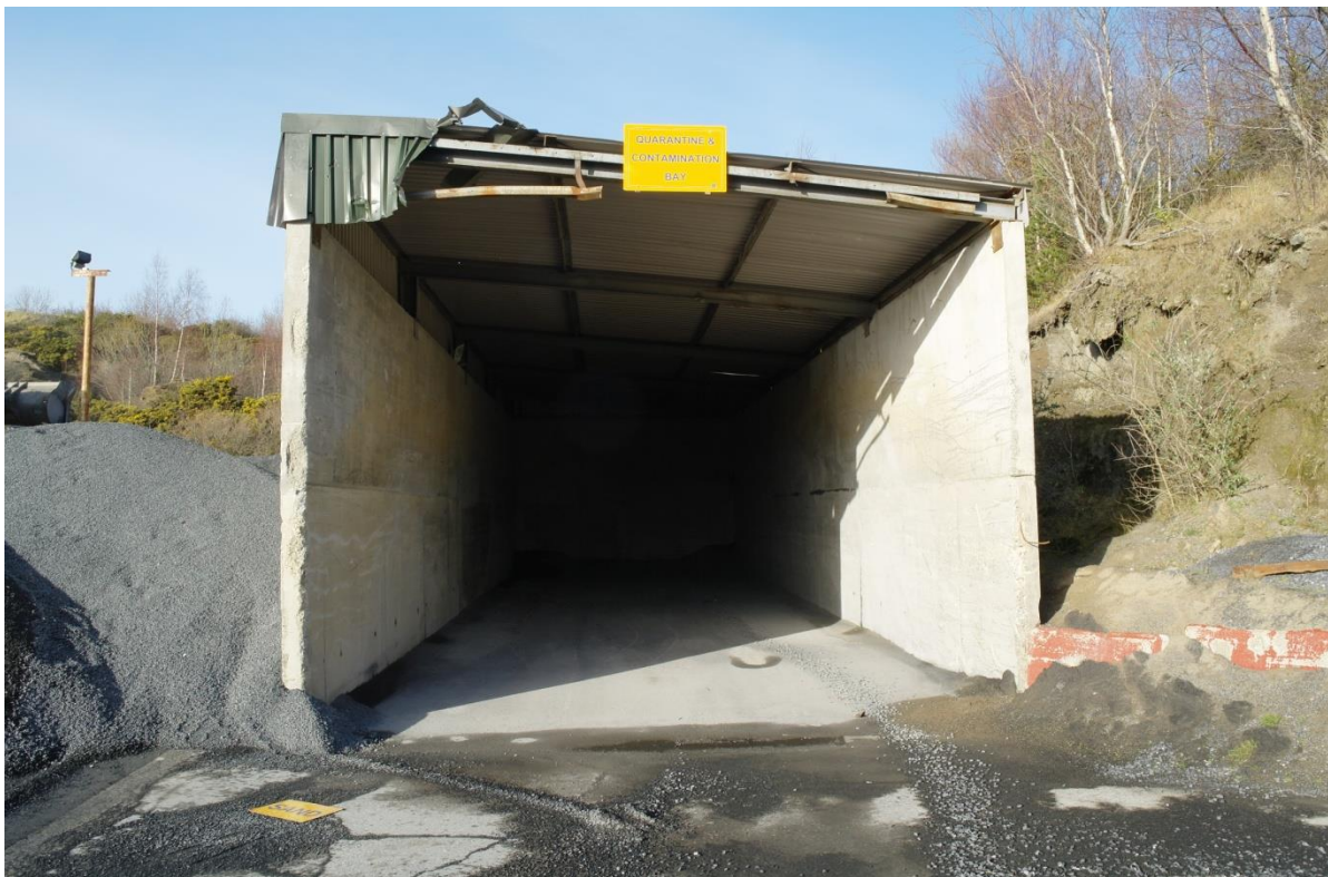
Photo 4 – Quarantine and Contamination Bay
