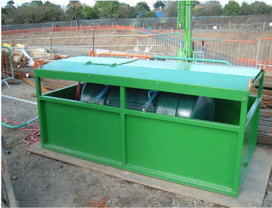
FIGURE D-6 TYPICAL BUNDED FUEL STORAGE AREA
