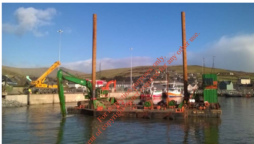
FIGURE D-4 ACN5 WITH A LONG REACH EXCAVATOR
