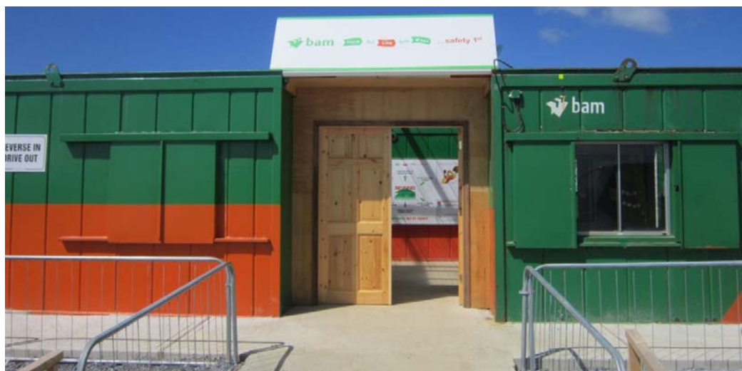
FIGURE D-9 TYPICAL SITE COMPOUND SET UP WHICH WILL BE USED ON THE BANTRY PROJECT
