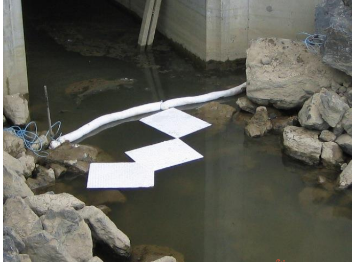
Photo 2: Spill kits located in diesel storage and refuelling area
