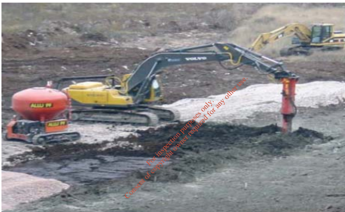
Figure 8: Dredge material being treated using the Allu treatment system
