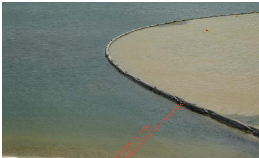
Figure 7.a: Environmental Silt Cutains used for the dredging operations
