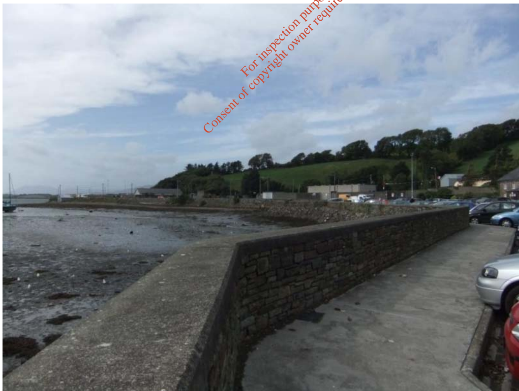
Plate 2.2 View from Public Car Park of Inner Harbour
