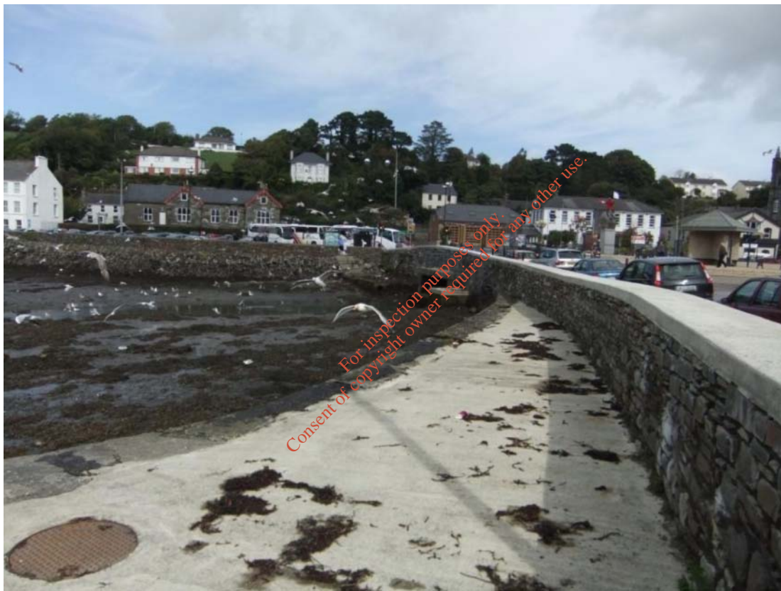
Photograph 2.7 Culvert Discharging to Harbour
