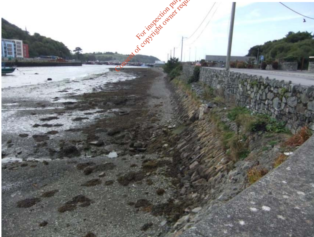
Plate 2.6 View of Northern Embankment
