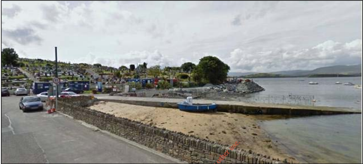
Plate 3.5 Slipway and boat storage facilities at Abbey Site
