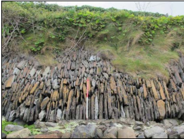
16. View looking at base of revetment along the north shore, showing the distinctive edge-set stonework that is seen in many of West Cork's small harbours
