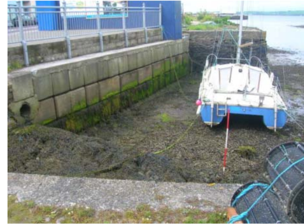
Newly built blockwork covering former area of slipway
