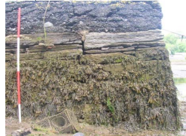
Exterior of west slip showing stonework and external batter
