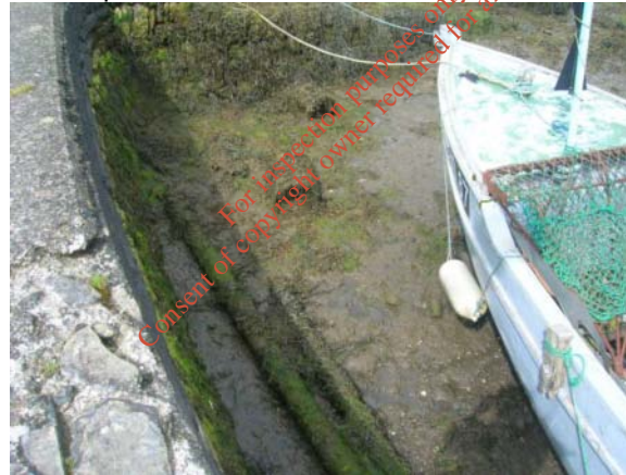
Detail showing curvature of stonework and internal batter
