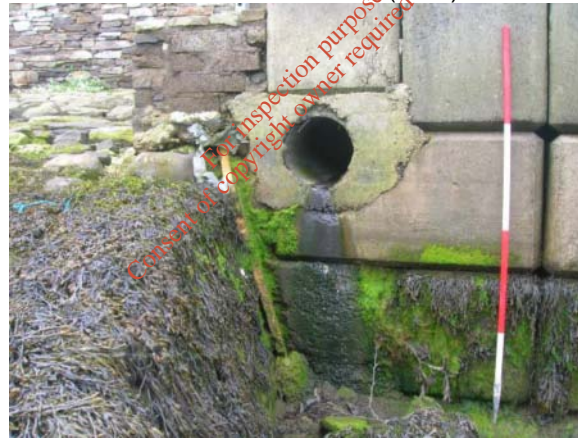
Detail showing nature of new build onto older stonework
