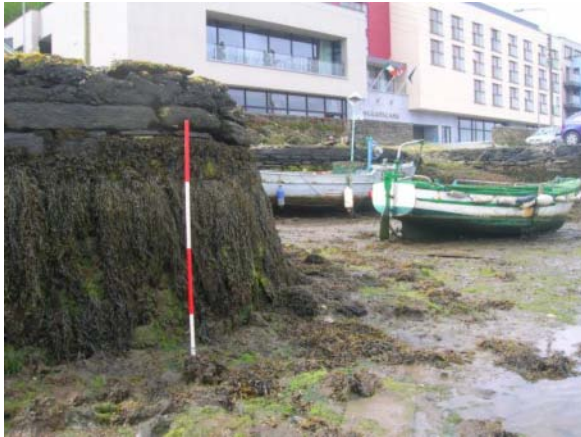
Exterior of east slip
