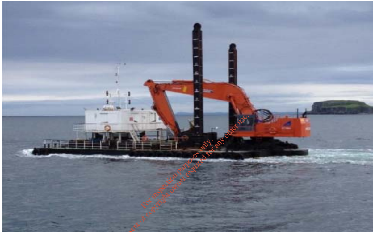
Figure 5: The Aoibheann Dredger which will be utilized for the dredging works
