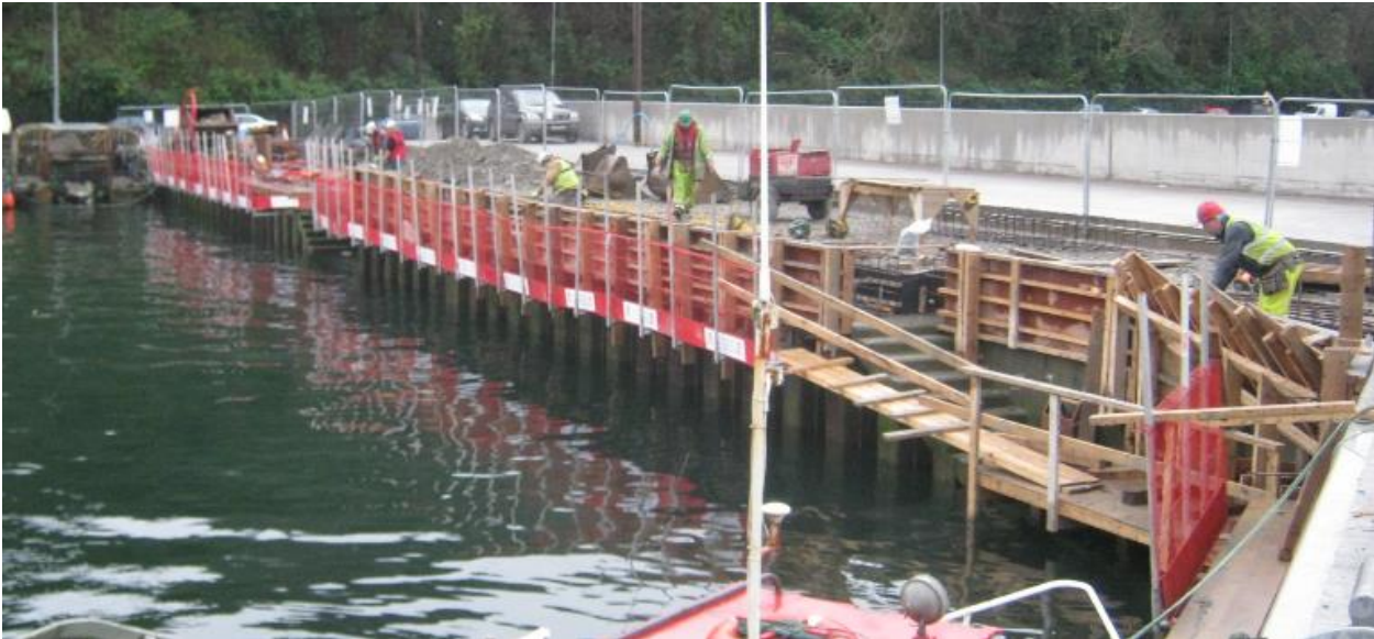
Picture: Temporary Walkway Provided on Previous BAM Marine Project
