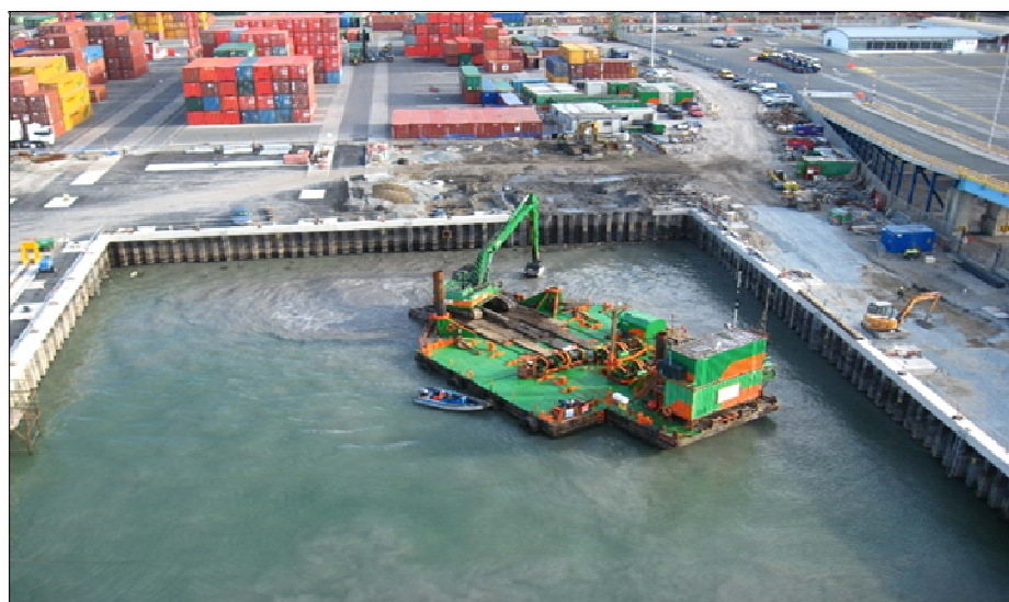
Figure 4: Bam Plant dredging in Dublin Port
