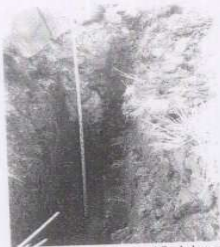
Trial Pit No. 1 – Material excavated to 3.4m below ground level
