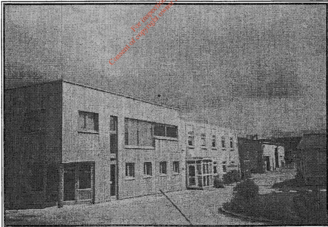
PHOTOGRAPHIC VIEWPOINT 4 - VIEW EAST TOWARDS SITE ENTRANCE
